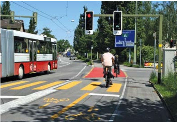
Figure 21. Two-way cycle path in Winterthur, Switzerland.
